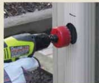
Drill hole in downspout
